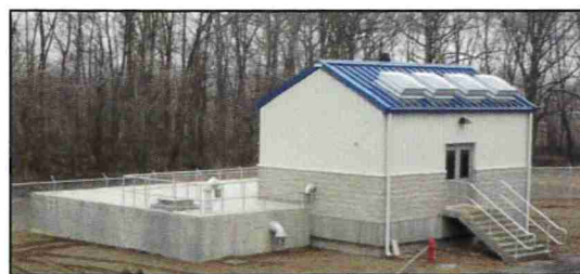
High Service Pump Building & Clearwell
