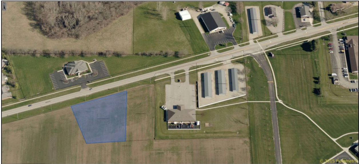
Figure 3. Marker Road site
